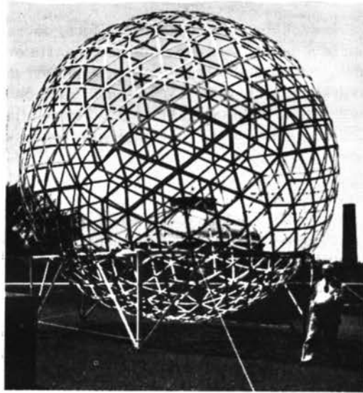
Geoscope at Cornell University School of Architecture, 1952. 20ft diameter
