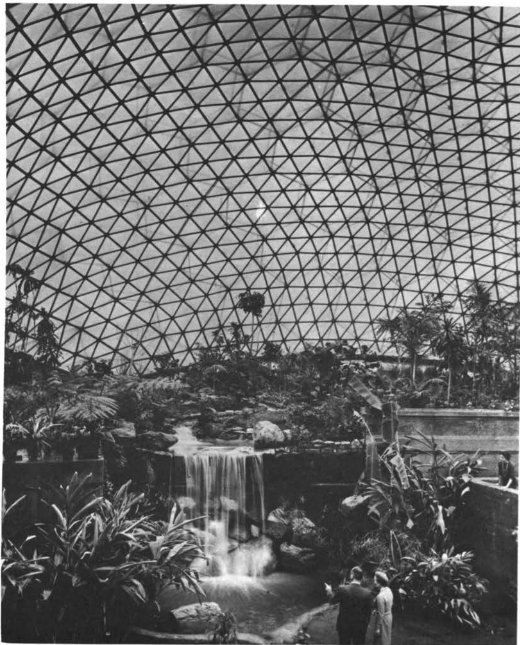
(S-13-30) To be able to control the geodesic Climatron's environment locally it maintains great differences in humidity and temperature at many points in the garden. Now in use for 3 years its acrylic skin has never required washing.
