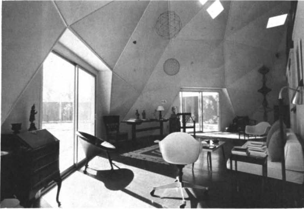
(C-11-25) This is the inside of my own home in Carbondale, Illinois. We live in a domical geodesic structure.
