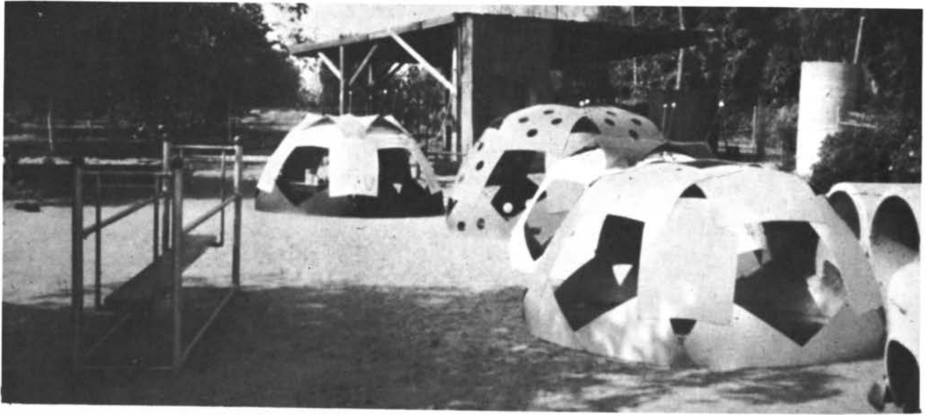
(P-20-1) This is just a children's playground with some small geodesic domes. Note that the pieces are of flat plywood bent into accommodation of a spherical structure. I call these geodesic plydomes.
