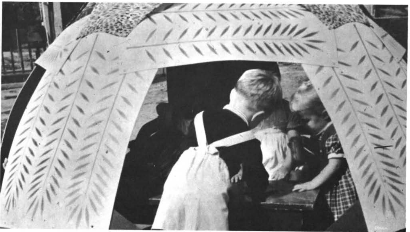
(P-20-4) The reason that I am showing this picture is because it is interesting mathematically that you can take a flat sheet of plywood and bend it simultaneously on five cylindrical axii. You can bend each of its four corners and you can also bend it in its middle and it thus becomes a spherical diamond, or a pair of compound curvature triangles.
