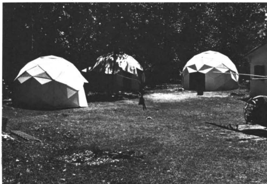
(M-32-18) These are some more foam core paperboard geodesic domes made by Monsanto Chemical Company, installed by the United States Peace Corp at Puerto Rico. I have had some of those paper domes go through hurricanes. They have to be tied down so that they won't blow away. They have to have some light wooden reinforcements inside their top sections to take full snow loads. Repainted every two years they will last for years.
