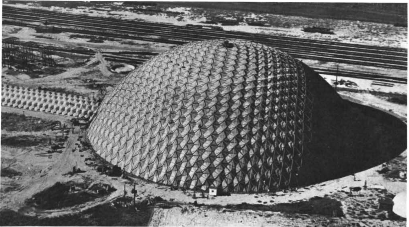
(U-2-75) another one of the 384 foot diameter domes at Woodriver, Illinois.
