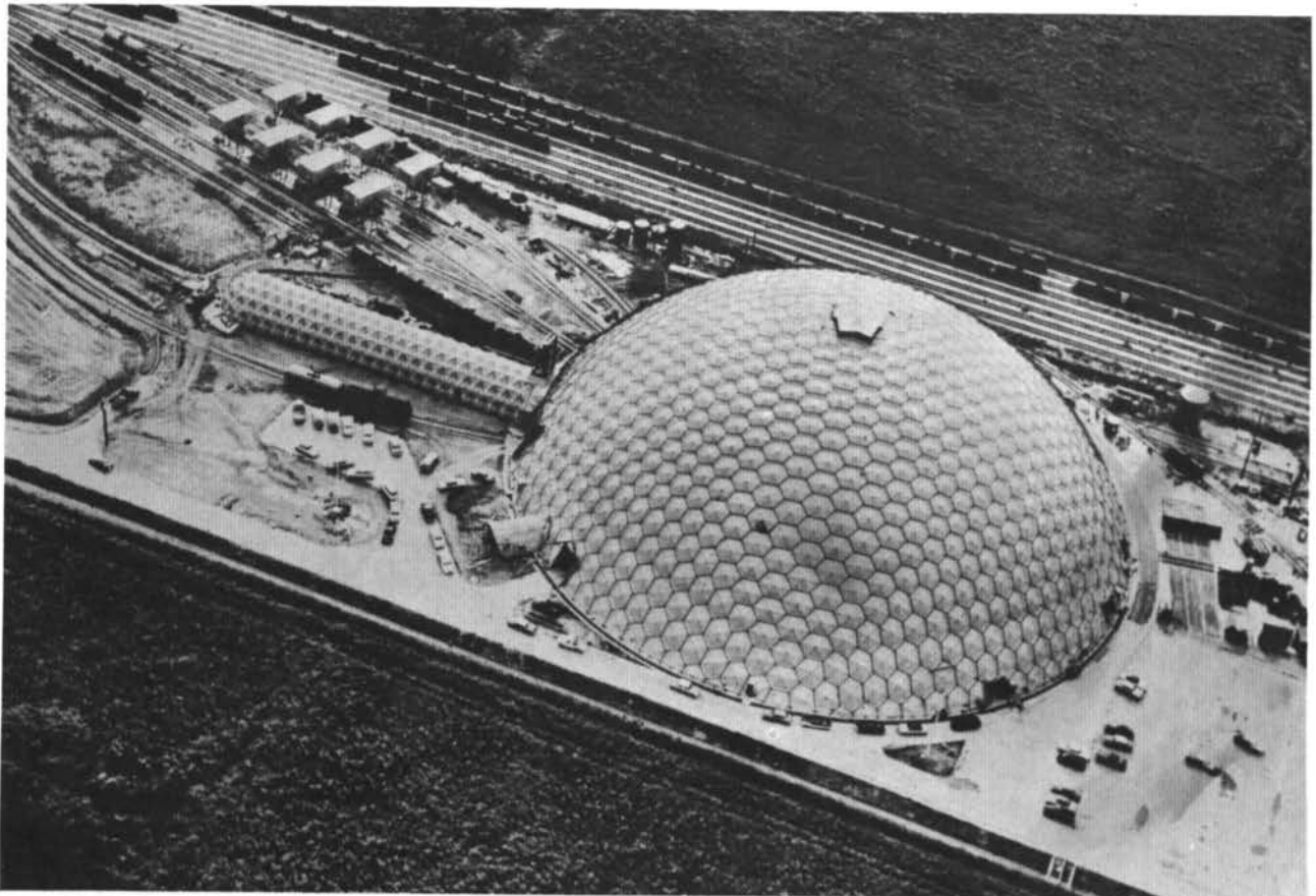
(U-2-71) This is in Baton Rouge, Louisiana, 1959. It is a geodesic dome 384 feet in diameter, made out of sheet steel suspended from a steel tube frame. It was put up by my licensee the Union Tank Car Company. The
