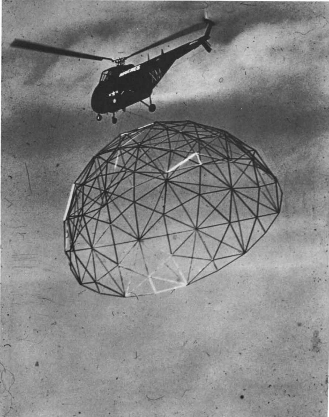
(M-8-16) The large helicopter carries the three-helicopter hangar away at a 60 knot speed. This was back in 1954.
